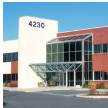
Crums Mill Professional Office Complex
